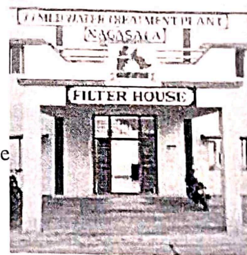
Figure 1: Water treatment plant, Nagasala
