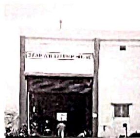
Figure 9 Clear water pump house
