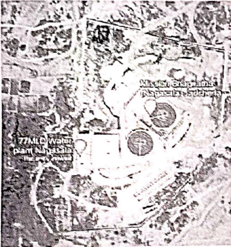
Figure 3. Nagasala Water treatment plant
